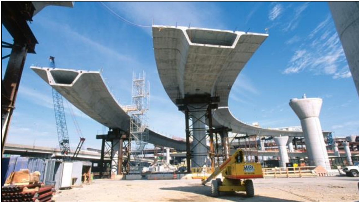
Figure 3-4 Concrete box girder bridge, location: unknown. www.shanghaimetal.com
