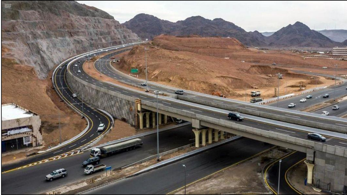
Figure 3-14 Composite overpass in Al Madinah, Saudi Arabia. www.Constructionweekonline.com
