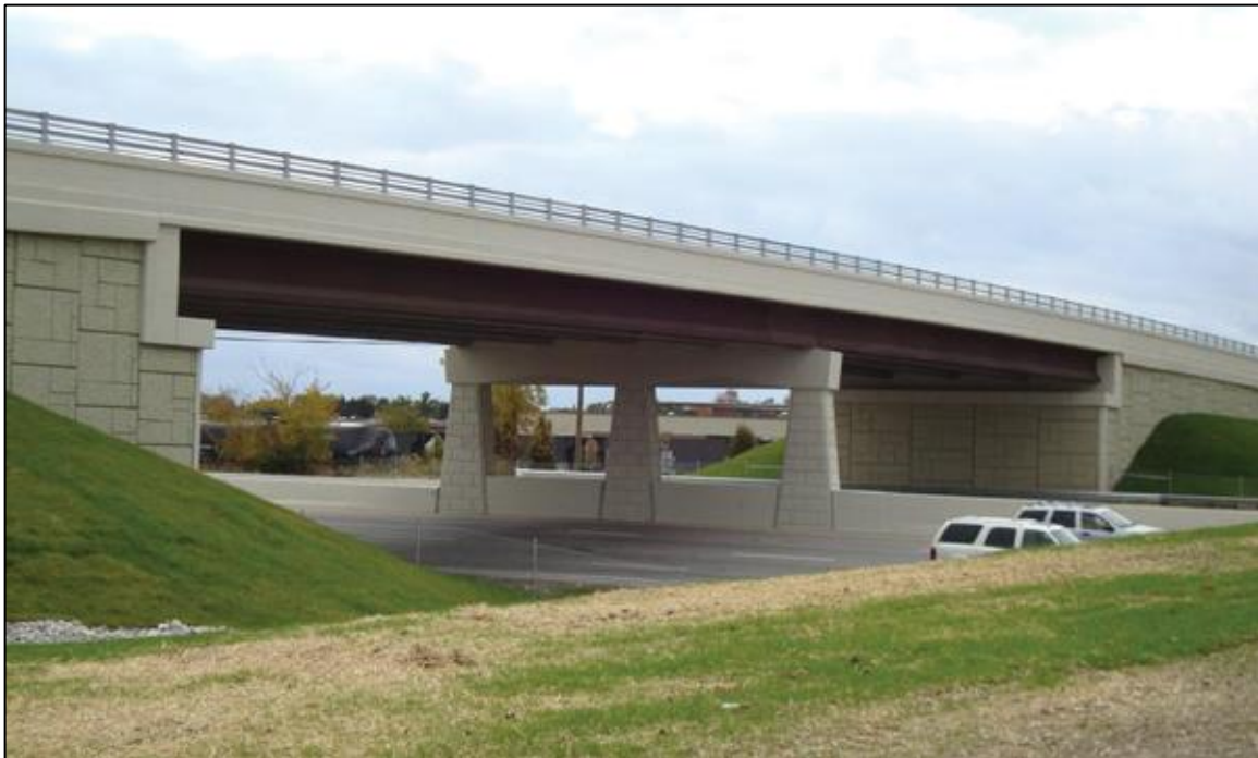
Figure 3-3 Beam Bridge example, location: unknown. www.nbmchw.com
