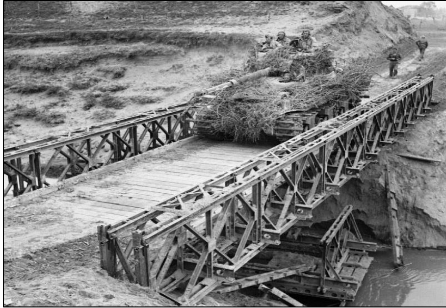
Figure 3-10 Heavily camouflaged Sherman tank crosses a Bailey bridge over the River Santerno near Imola, 12 April 1945. www.thinkdefence.co.uk
