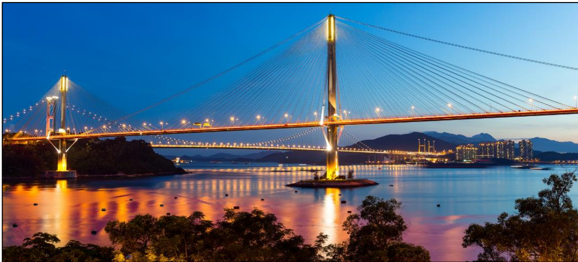
Figure 3-5 Ting Kau Bridge in Hong Kong. www.alamy.com
