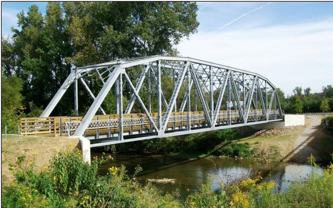
Figure 3-7 Truss bridge, location: unknown. www.usbridge.com
