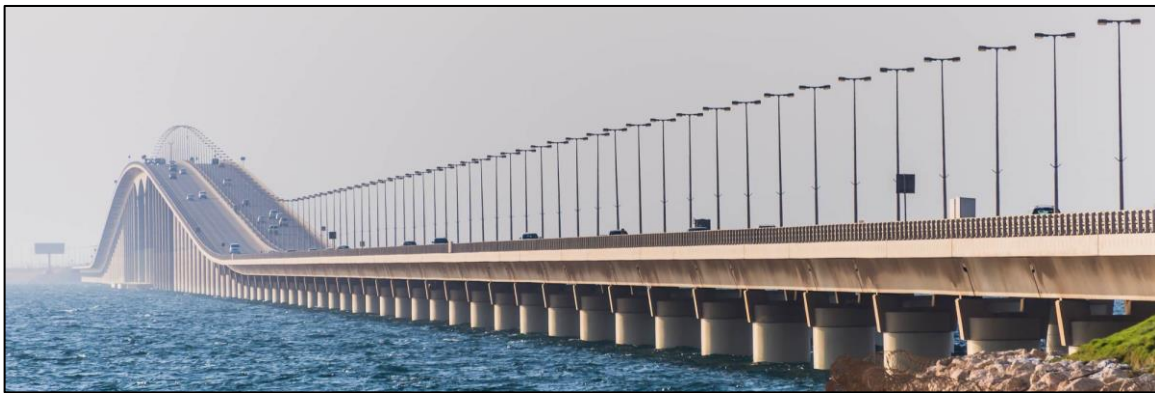
Figure 3-1 King Fahad Causeway Bridge. www.commercialinteriordesign.com
