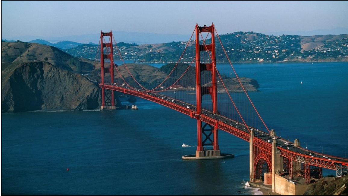
Figure 3-2 Golden Gate Bridge - California, USA. www.cnn.com
